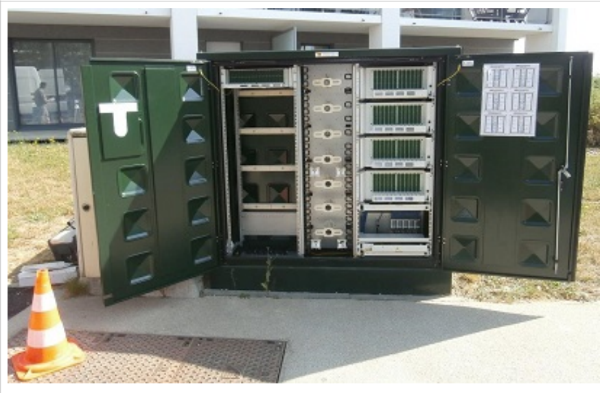
A French 'point de mutualisation'. These road-installed units typically connect 360 premises or as many as 1,000
